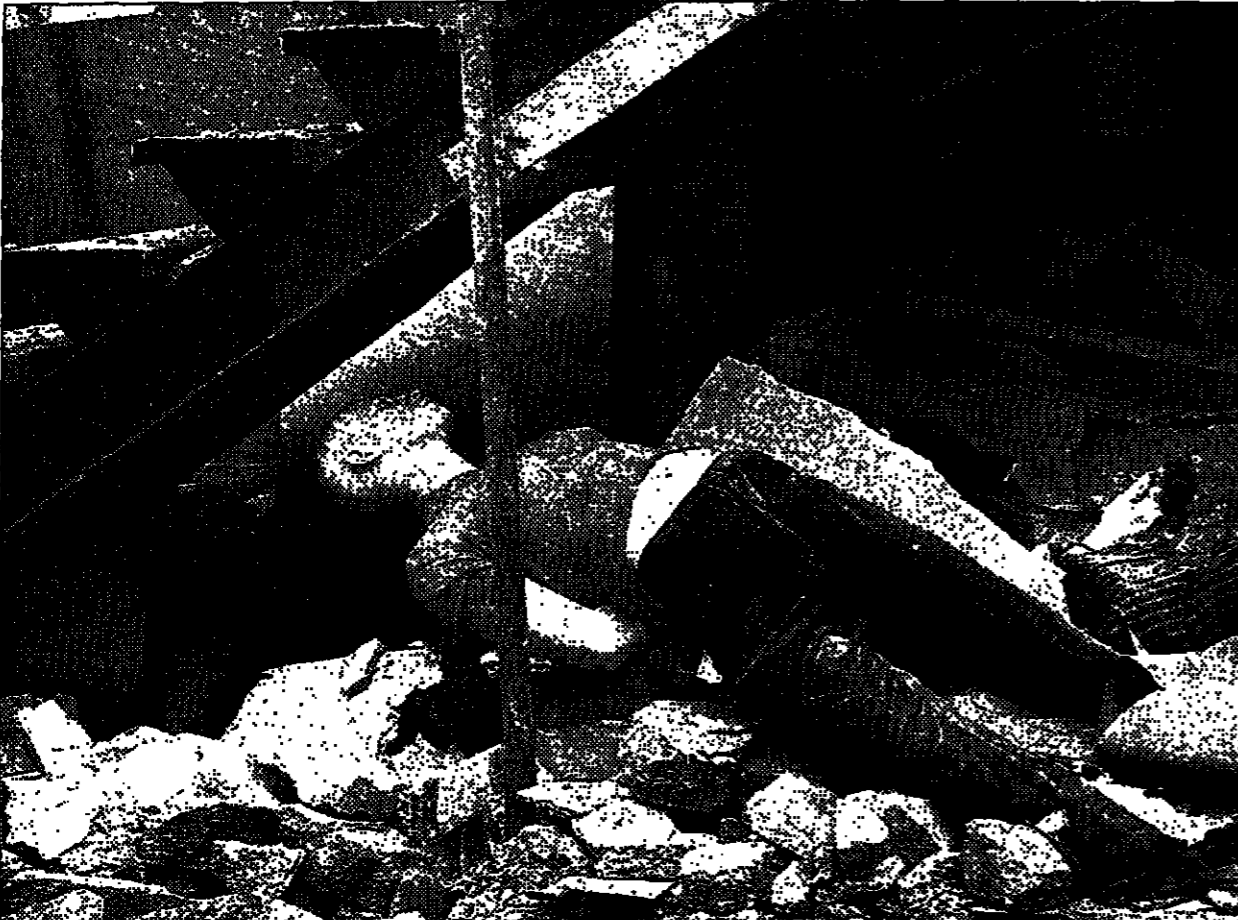
A broken mannequin lies in rubble still to be cleared from a battered building in Manchester. PHOTOGRAPH DON MCPHEE
